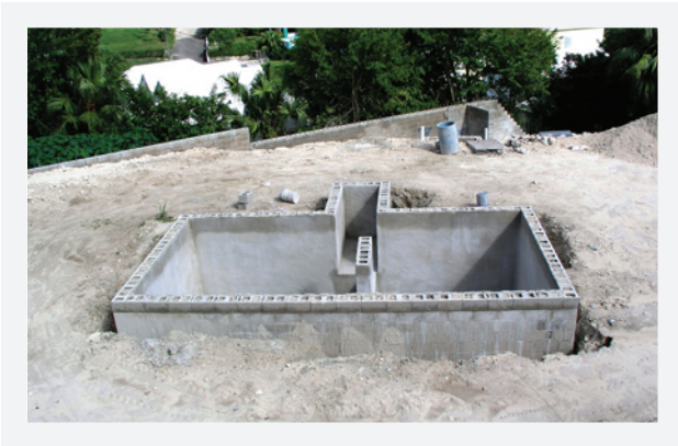
A typical Bermuda tank has a capacity of 13,500 Imperial gallons. Photo courtesy of Mark Rowe
