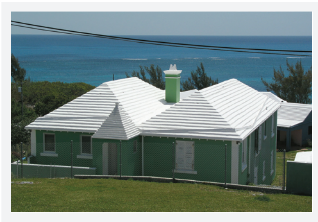
A typical Bermuda roof has a catchment area of 1360 square feet.
